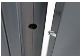
Fig. 37. Anti-burglary bolts (standard)
